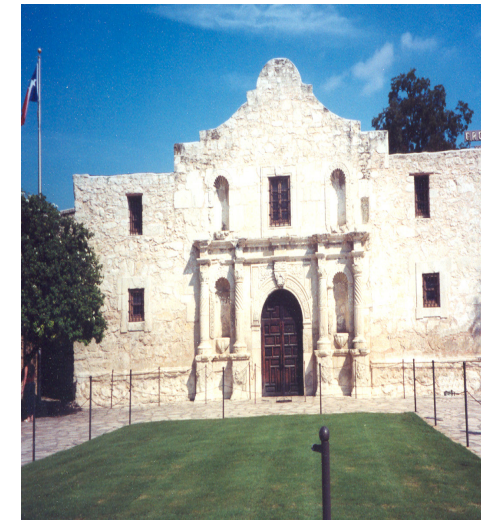
After the battle of the Alamo, the U.S. Army completed the roof on this building for the first time and repaired the famous “hump.”
